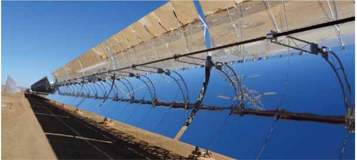
Figure 2: Parabolic mirrors with receiver pipes.
