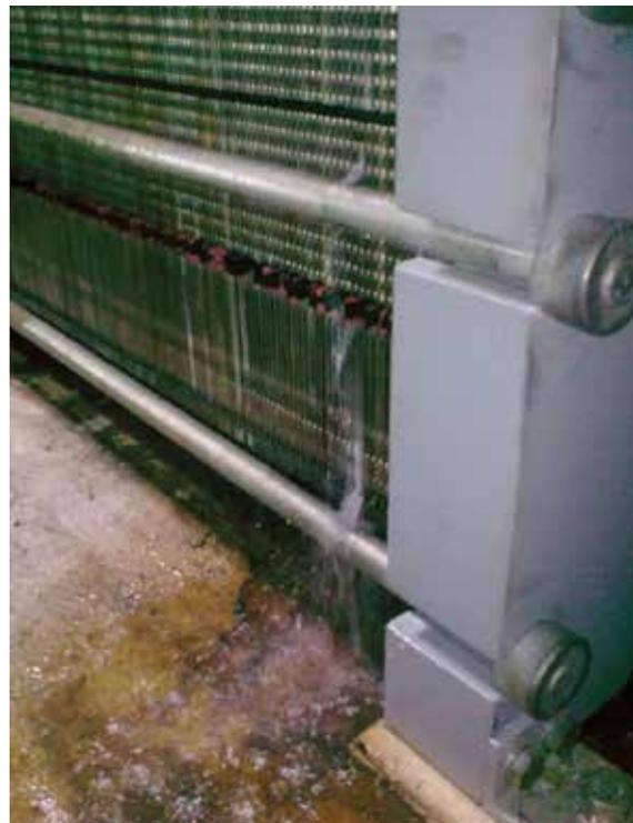
Figure 2: Partial view of the plate heat exchanger with a leak (Image: Siemens)
