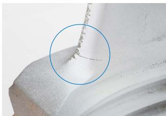
Crack in a steam turbine blade
